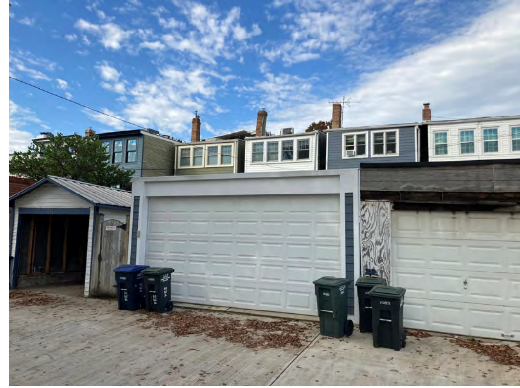
VIEW LOOKING SOUTH IN ALLEY
