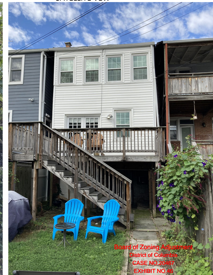
EXISTING REAR FACADE
